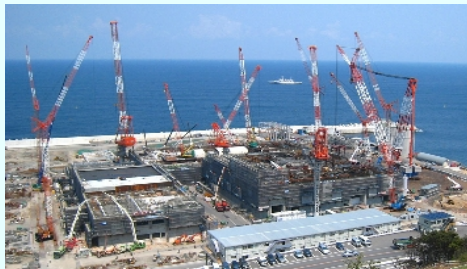
Chugoku Electric Power CO. Shimane-3 (Under construction) (NSSS and BOP)
