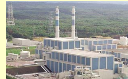
Hokuriku Electric Power CO. Shika-2 (2006) (NSSS and BOP)
