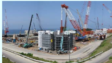
Electric Power Development CO. Ohma (Under construction) (NSSS (Full MOX ABWR))
